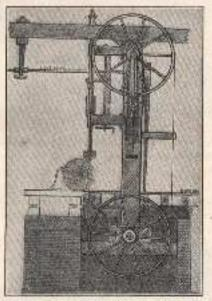
Fig. 53.-One of the first hand-saw machines.
