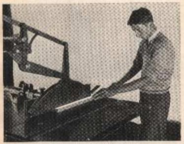
Fig. 39. Correct position at circular saw.
