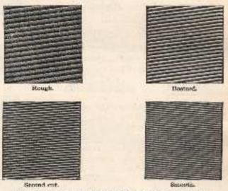
Fig. 82.-Four main graduations of single-cut files (12 inch size).
